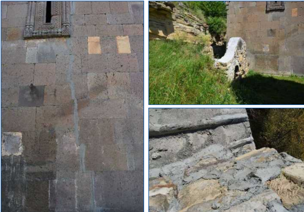
Figures A1.56a,b,c: Use of cement in the reconstruction and repair work at Tiri Monastery, 2016. ©Blue Shield Georgia.
