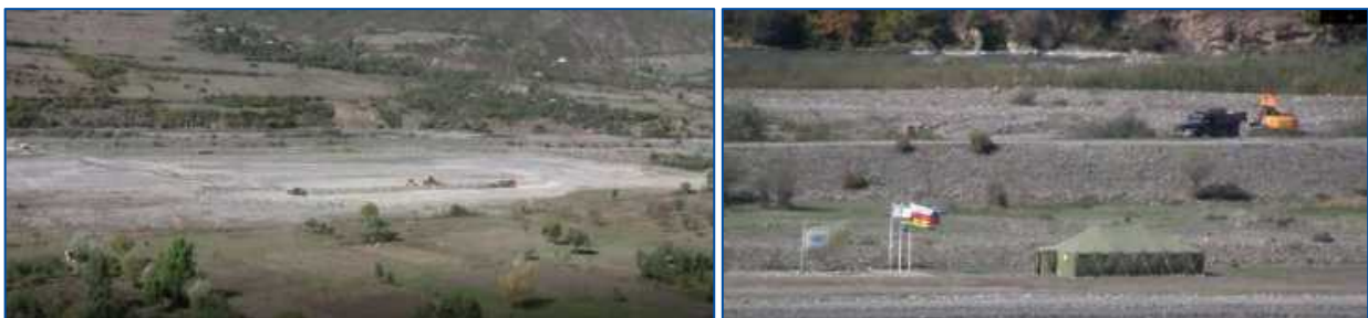
Figure A1.32, A1.33: Historic Orchards of the palace being bulldozed (2010) © Didi Liakhvi Valley Museum-Reserve
